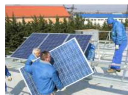
installation of solar systems
